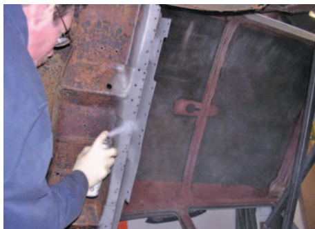
Photo #10: The entire flange was then coated with a weld-through primer.
