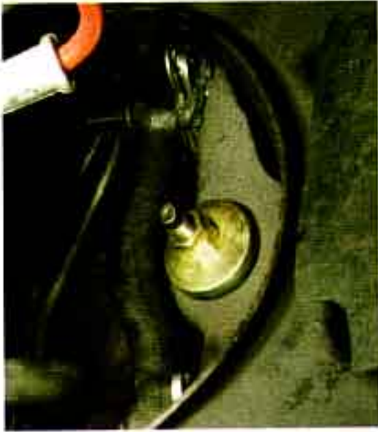
Photo #15: The top shaft of the shock absorber mounts to the top of the frame with a rubber grommet, washer and nut.
